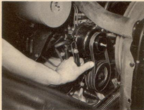
Tension on all belts is 3/8" — as in this belt from pressure pump (lower) to centrifugal governor (on DS-19).
