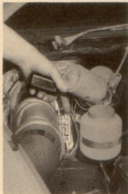
Fuse box (right side)
